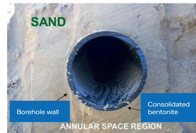
Figure 32. HDD installed 200mm diameter duct excavated 1 year after installation. Ariaratnam & Beljan (2005).
