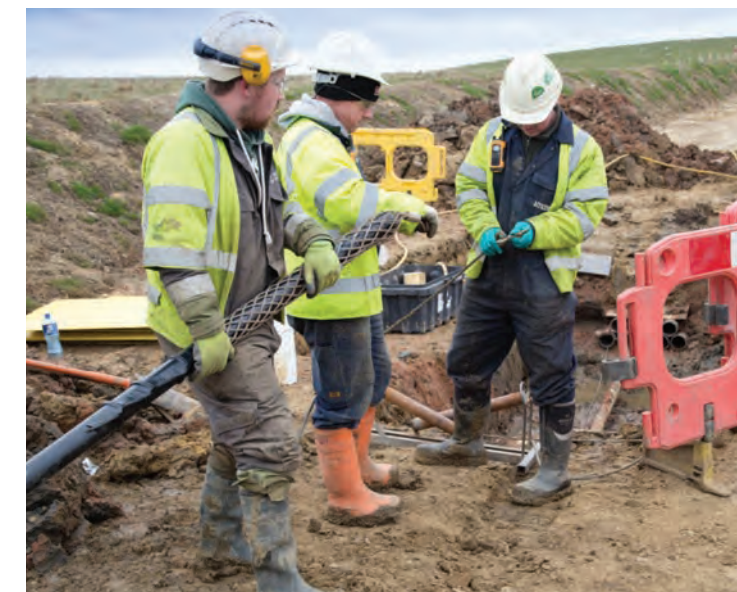
Cable pulling preparation
